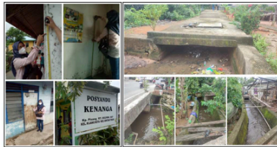
Fig. 2 Flood Inundation Height Location, Documentation 2021
