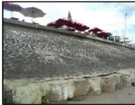
Figure 2. SeawallCrumblingon Canggu Beach, Bali,Indonesia (Nalarsih, 2016)
